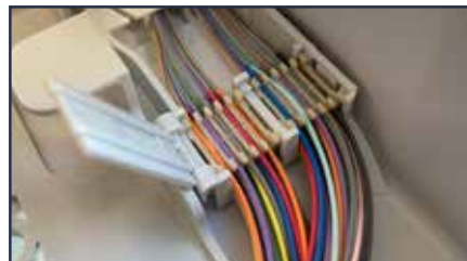
Foam and lock to fix pigtails
